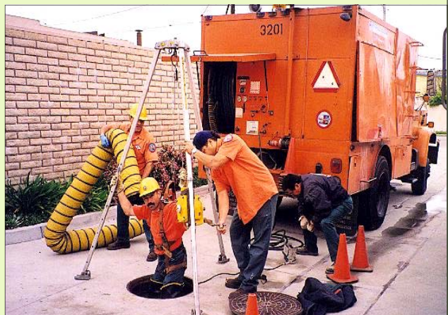
Sewer Crew at Work
